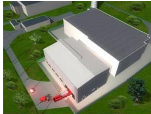
The Dry VVER-440 Spent Fuel Storage in Kozloduy NPP (Bulgaria)
